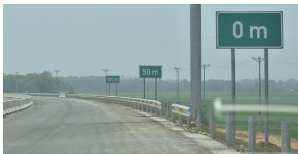
Figure 4: Safe distance signboard on the Mai Son Expressway (Phạm Hải, 2024)
